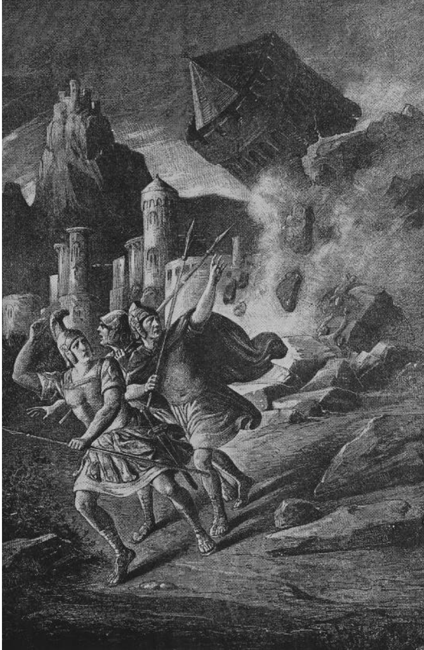
COLLAPSE OF THE TOWER AT GAMALA
