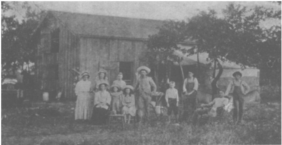
First building in the town of Bethany, Okla. This barn was the first home of the Jernigans after they moved to Bethany from Texas. Here is the family with some of the helpers.
